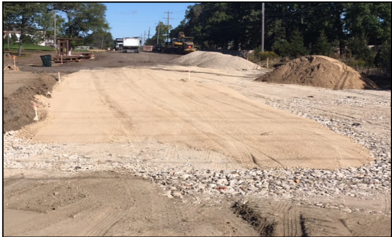
County H Facing North
