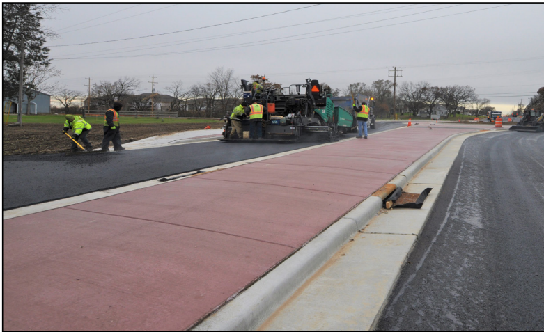
Paving operations facing north
