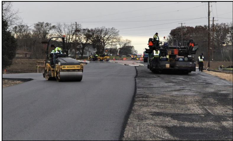
Paving operations facing north
